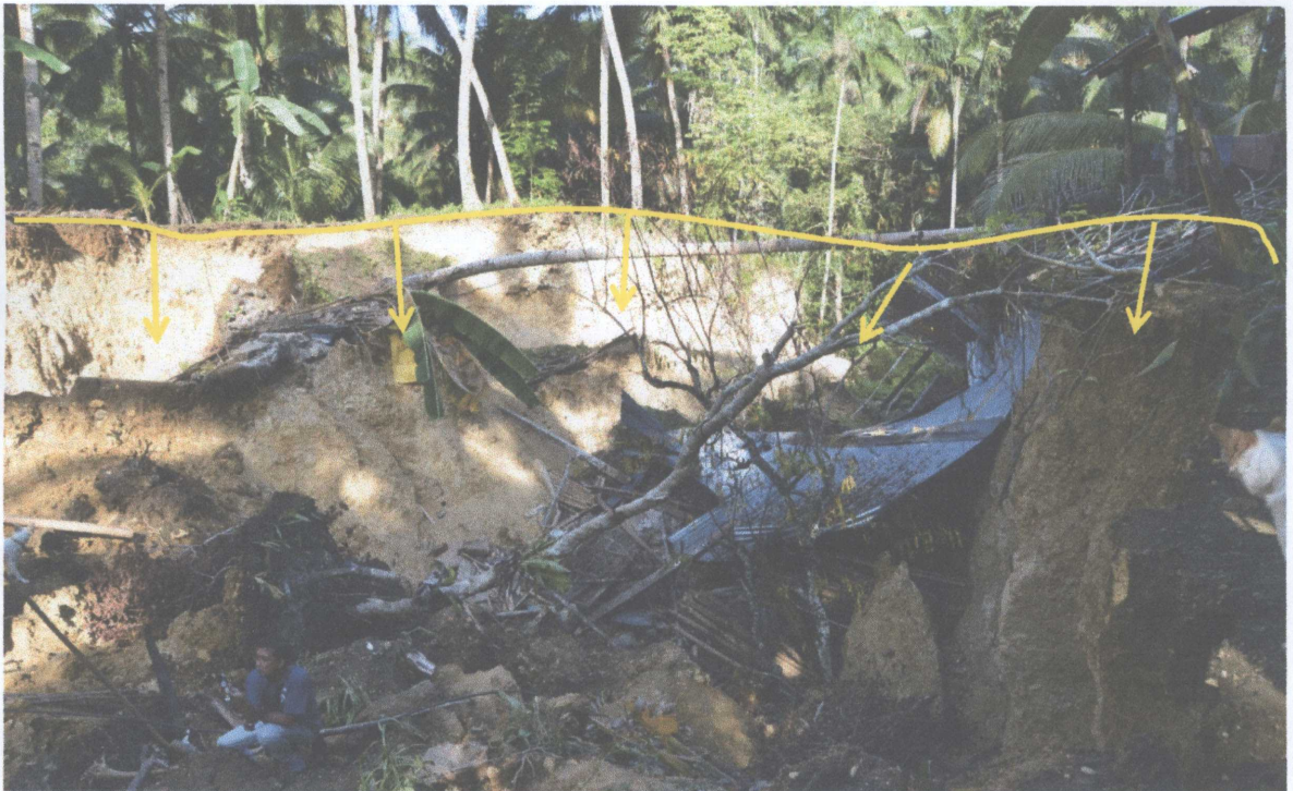
Sinkhole collapse in Antequera, Bohol due to October 2013 Bohol earthquake
