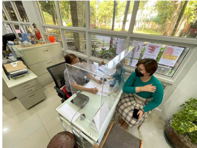
Figure 27. Installation of acrylic barrier in NAPWC Office to avoid transmission of COVID 19 between NAPWC employees and its clients
