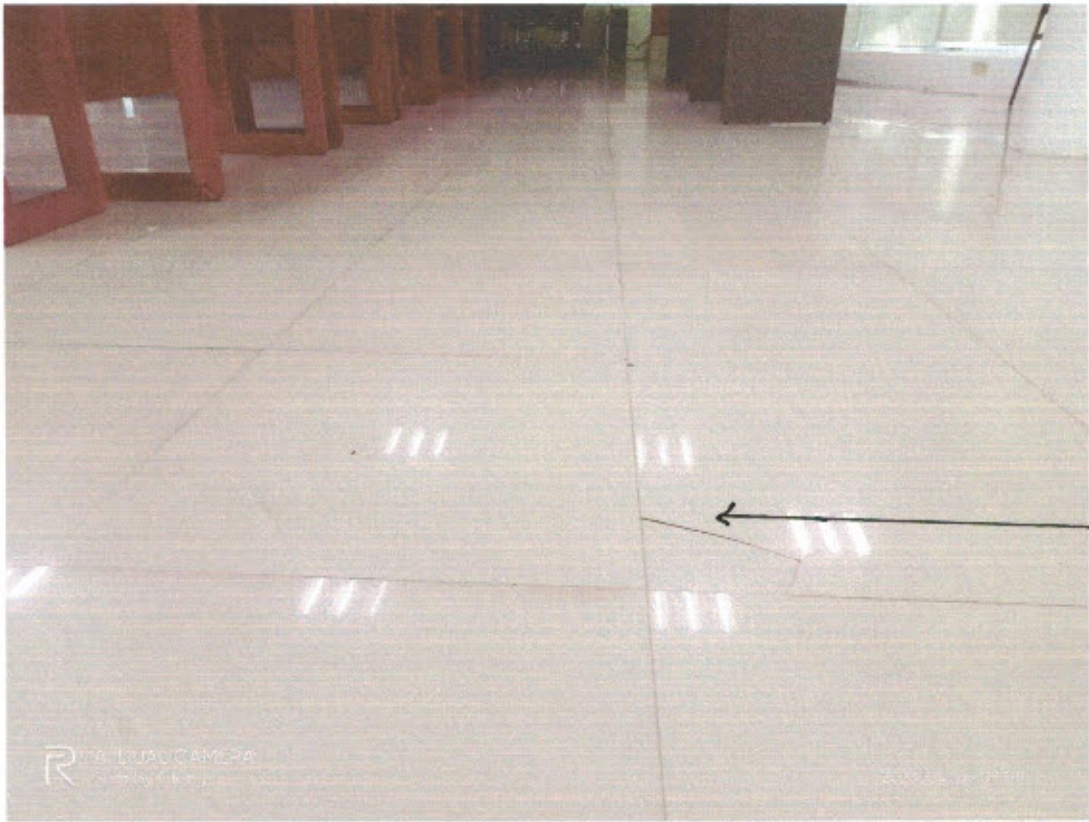
Existing floor tiles (sira-sira na)
